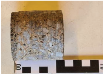
Foto 9: Bohrkern KRB 16 (Halle 3)
